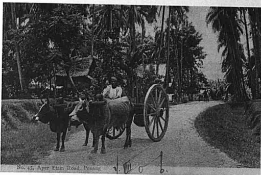
No. 45, Ayer Itam Road, Penang.
